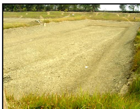
Pond bottom after top soil removal
