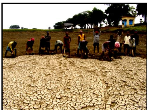
Top soil removal
