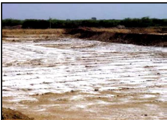
Lime applied on pond bottom
